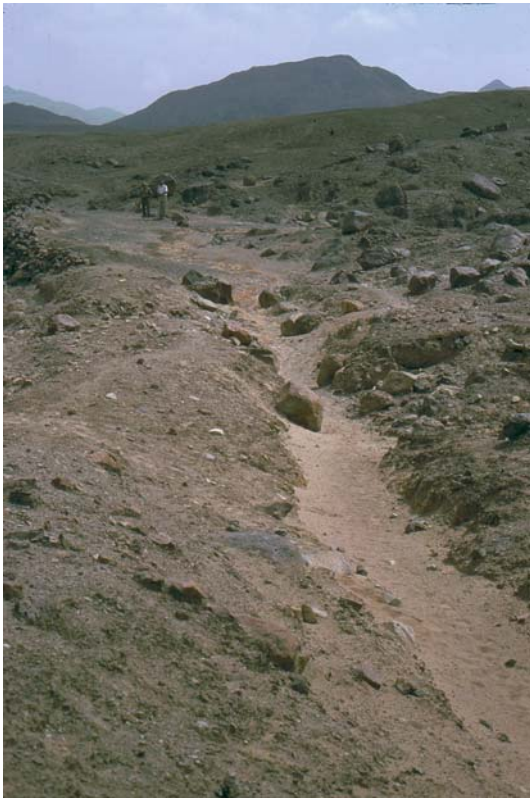
Water Management in Peru. Fig. 7 Unexcavated view of the hydraulic control structure upstream of the chute and the Hoya Hondada aqueduct; structure consists of opposing boulder pairs in the main channel separated by a 13.2 m distance. Photo by C. R. Ortloff.
